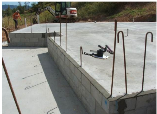
Figure 40 ARMOUR-THOR construction joint after casting
