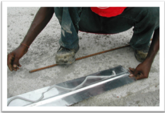
Figure 18 ARMOUR-THOR folded for construction joint
