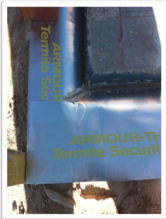
Figure 27 ARMOUR-THOR being folded into cavity where brickwork is at same level as concrete slab
