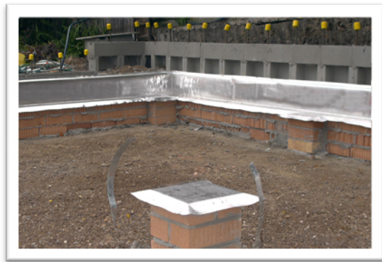
Figure 22 ARMOUR-THOR as pier cap
