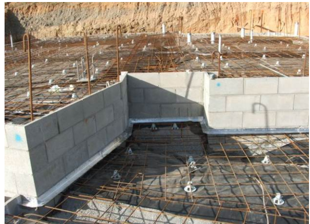
Figure 39 ARMOUR-THOR construction joint
