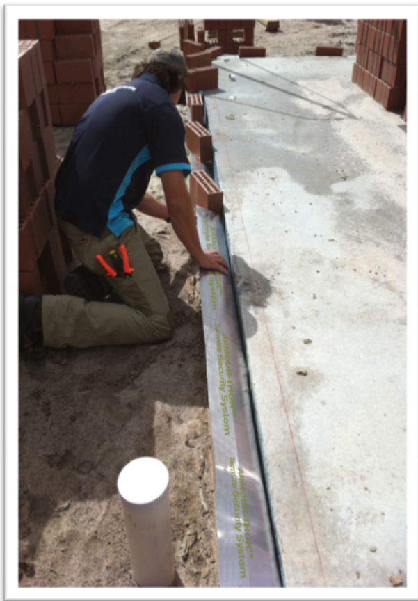
Figure 28 ARMOUR-THOR being folded into cavity where brickwork is at same level as concrete slab
