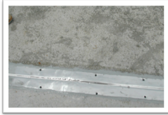
Figure 21 ARMOUR-THOR nailed and glued to slab. Nail heads to be covered with NOVITHOR Flexi-Gel
