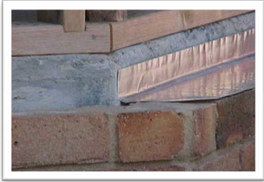
Figure 16 ARMOUR-THOR position in rebate application
