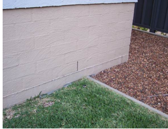
Figure 5 ARMOUR-THOR positioned between weep hole and first course of brickwork (creating 75mm inspection zone)
