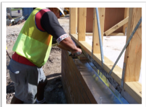
Figure 11 ARMOUR-THOR moulded to shape
