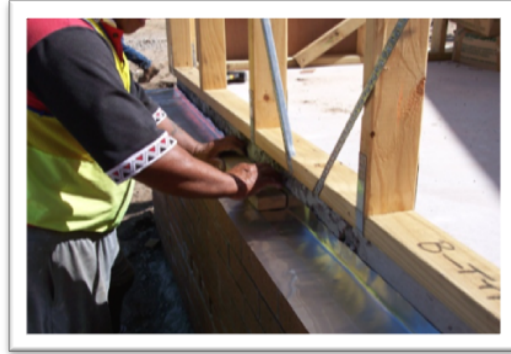
Figure 12 ARMOUR-THOR top edge folded over to form v-joint for application of NOVITHOR Flexi-Gel
