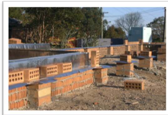
Figure 23 ARMOUR-THOR for perimeter bearer and joist and engaged pier application
