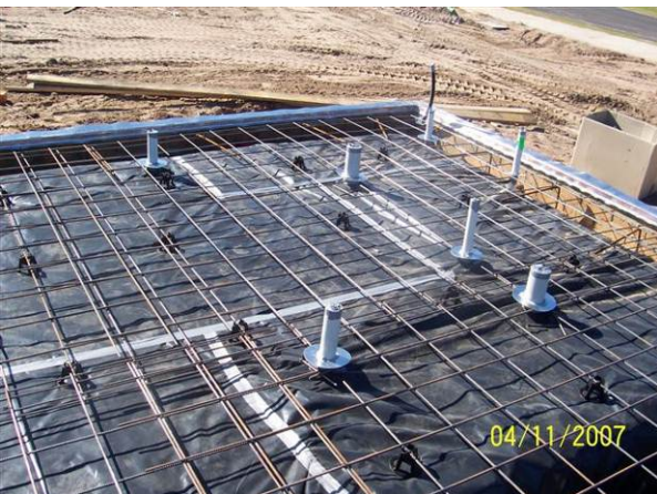
Figure 37 ARMOUR-THOR collars and perimeter casting
