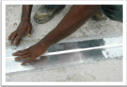
Figure 19 ARMOUR-THOR positioned on top of construction joint. NOVITHOR Flex-Gel being applied.
