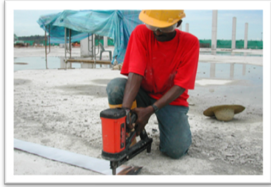
Figure 20 ARMOUR-THOR fastened to slab with nail gun
