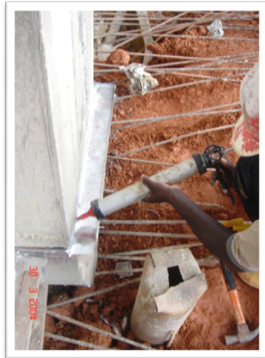
Figure 26 ARMOUR-THOR construction joint. NOVITHOR Flexi-Gel being applied to the v-joint in the ARMOUR-THOR.
