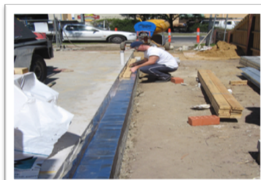
Figure 12 ARMOUR-THOR top edge folded over to form v-joint for application of NOVITHOR Flexi-Gel
