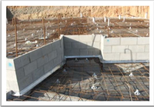
Figure 24 ARMOUR-THOR attached to concrete slab edge and cast into concrete slab as construction joint
