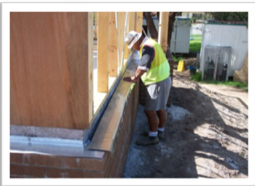
Figure 10 ARMOUR-THOR folded over brickwork
