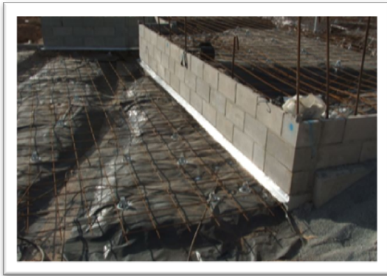
Figure 25 ARMOUR-THOR attached to concrete slab edge and cast into concrete slab as construction joint
