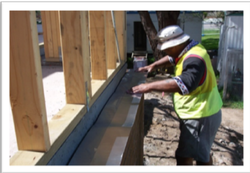
Figure 9 ARMOUR-THOR being positioned
