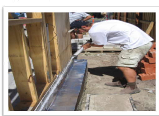
Figure 14 NOVITHOR Flexi-Gel applied to v-joint
