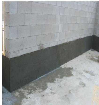
Figure 6 NOVITHOR Cementitious Parge minimum 4mm thick applied over brick work in step down area between upper and lower concrete slabs
