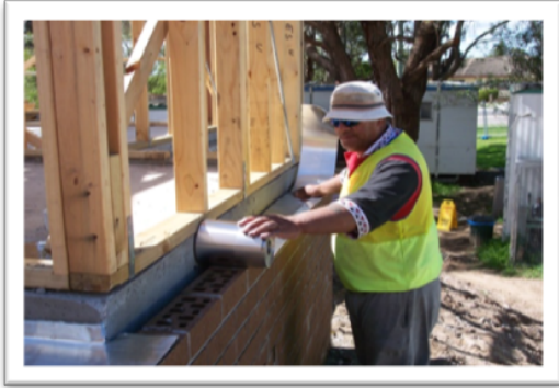
Figure 8 ARMOUR-THOR being rolled out
