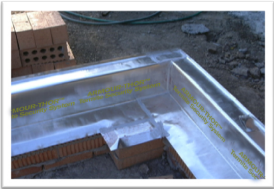
Figure 17 ARMOUR-THOR bearer and joist application
